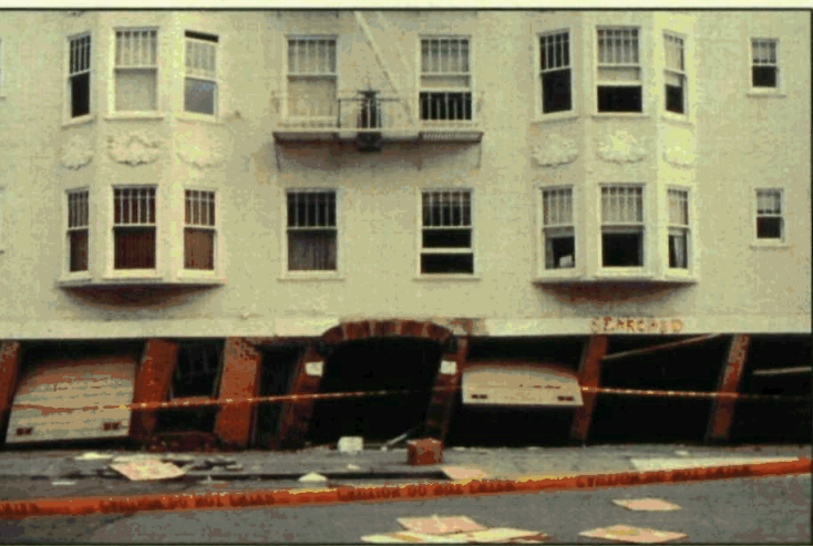
This "soft"-first-story building failed partially during the Loma Prieta earthquake. In some buildings nearby, the first floor was totally destroyed.
