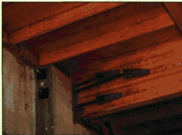
Extra ties can readily be added to strengthen older tilt-up buildings.
