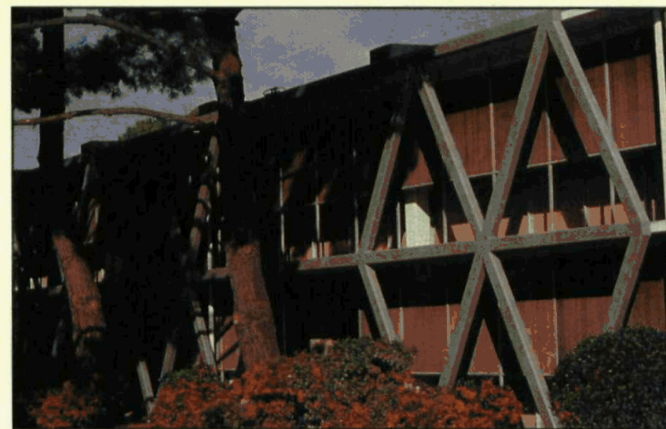
This diagonal steel frame effectively braces a concrete frame building housing U.S. Geological Survey employees.
